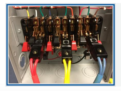
Install the blue C phase duckbill into C current return on the test switch. Make sure the black side of the duckbill connector is facing towards the meter.
