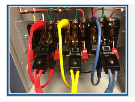
Install the blue current jumper from the bottom of the C phase current return terminal to the top of the C phase current input terminal.
