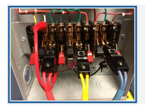
Install the red current jumper from the bottom of the A phase current return terminal to the top of the A phase current input terminal.
