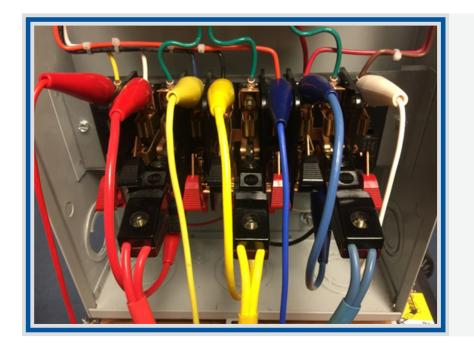
Connect the fused leads to the top side of A, B, and C voltage terminals. Connect the neutral wires to the top side of the neutral terminal in the test switch.
