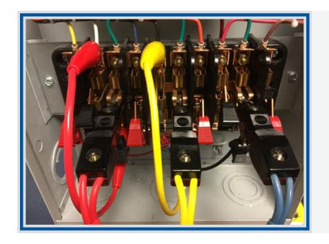
Install the yellow current jumper from the bottom of the B phase current return terminal to the top of the B phase current input terminal.
