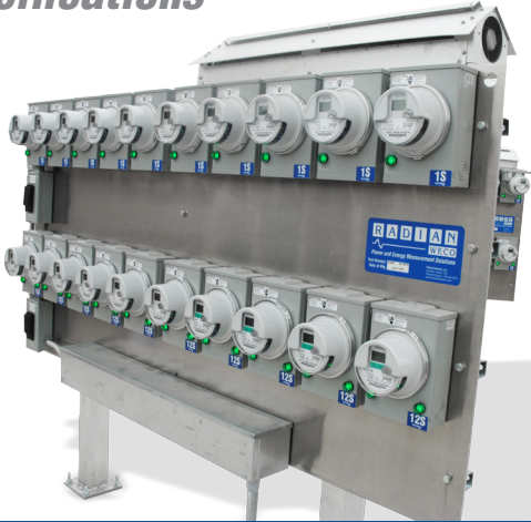
Radian Custom Built WECO Meter Farm WECO AMI Meter Farm
