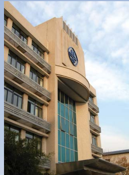
The location of the new Radian Research Calibration and Repair Center China (Inside China National Metrology Institute)
